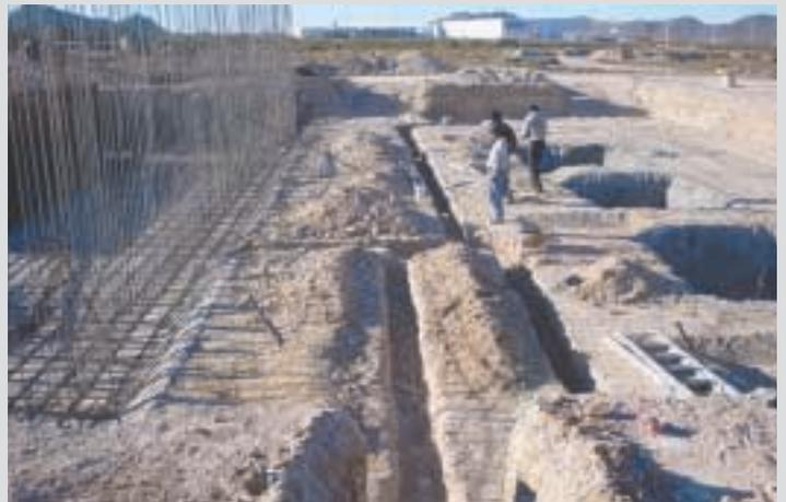
work in progress, excavation works for grounding system
